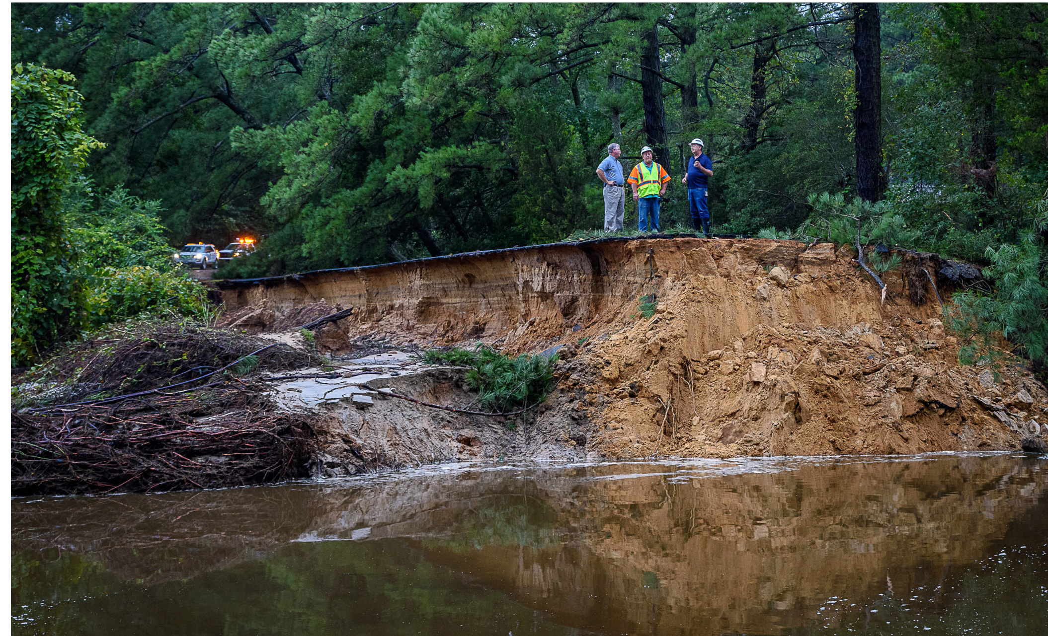
Road Washout in Belle Haven, VA
